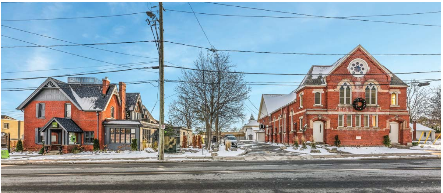
Figure 1: Photo of Existing Site, Mountain Street Frontage
