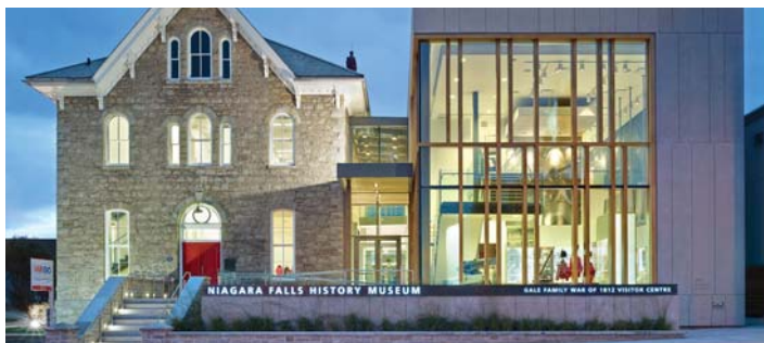
Figure 15: Connection to New Proposed Residential Mass - Niagara Falls History Museum, Niagara Falls ON
