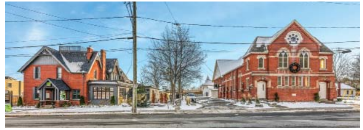
Figure 6: Photos of Existing Buildings on Site
