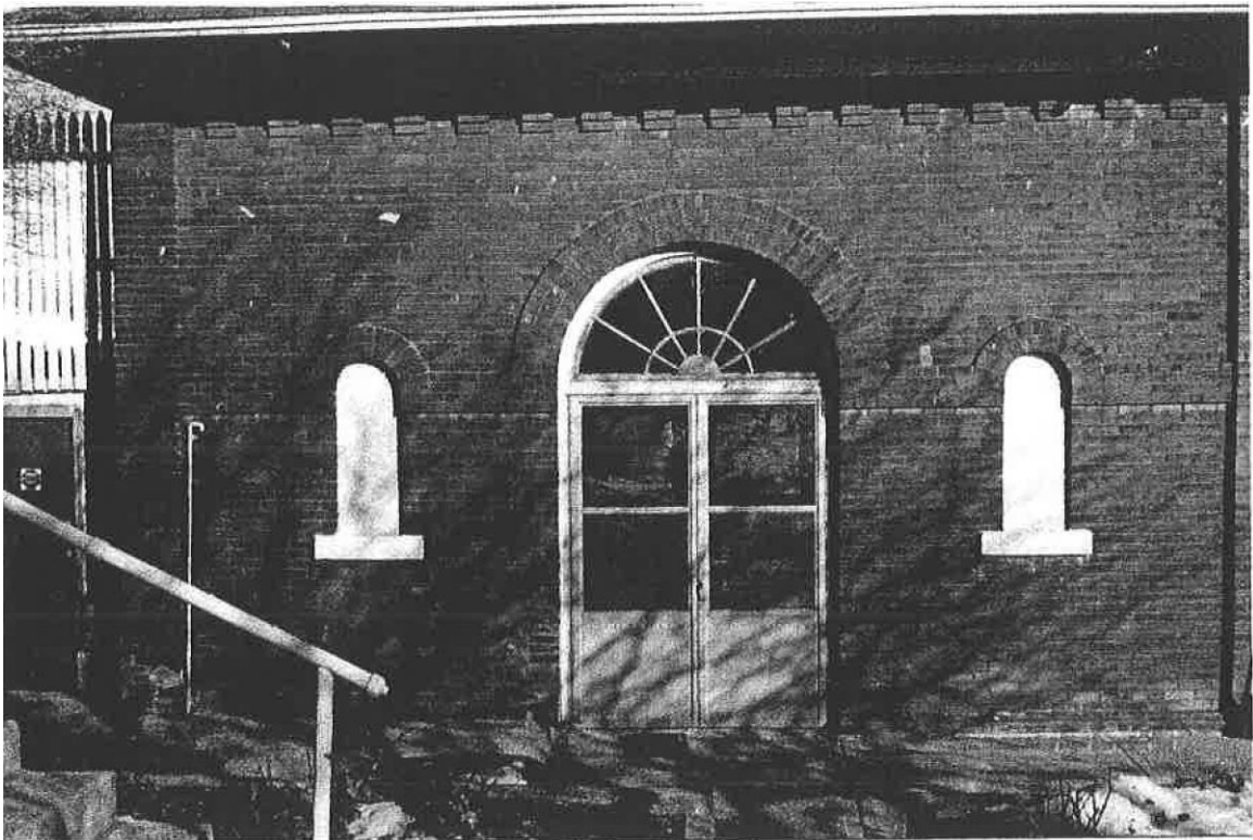
3. exterior, south elevation of west section
