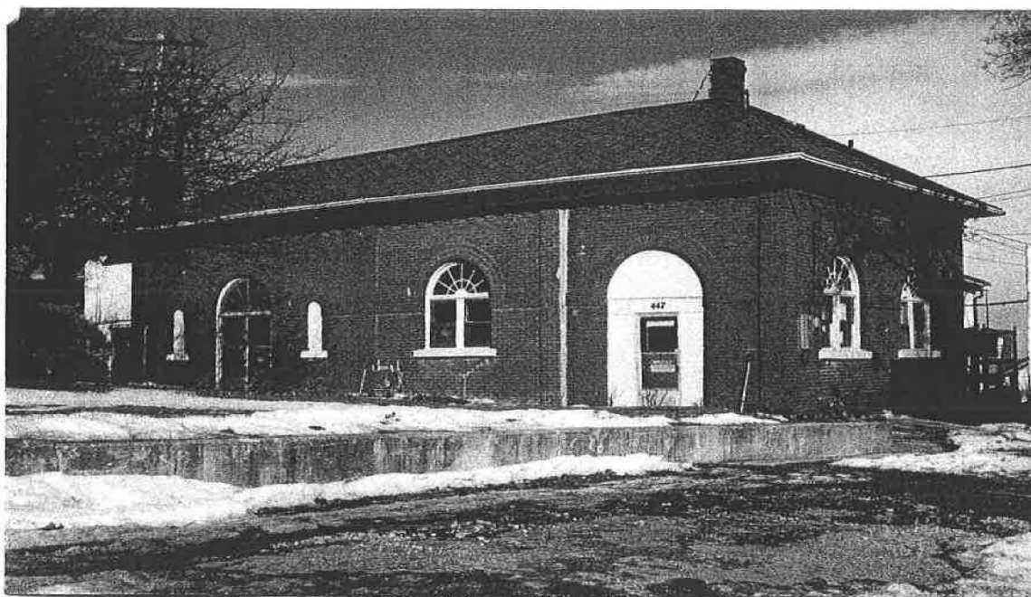
Exterior from Southeast
