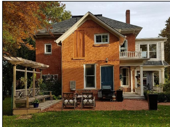
Figure 26: 224 Main Street East, looking north towards patio at the rear of the existing building
