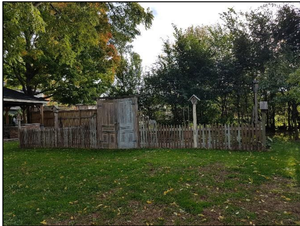
Figure 25: 224 Main Street East, looking east and showing a fenced garden in the rear yard
