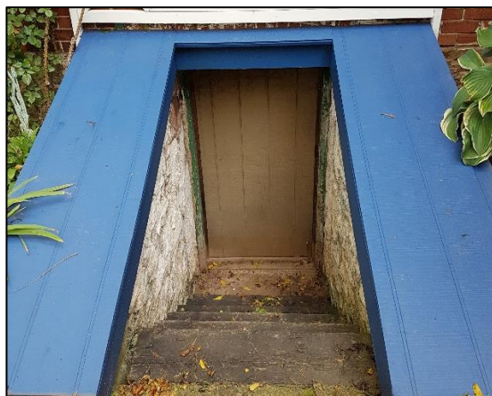
Figure 37: 224 Main Street East, showing cellar entrance on rear elevation
