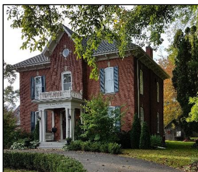
Figure 3: 224 Main Street East, looking south (ASI 2018)
