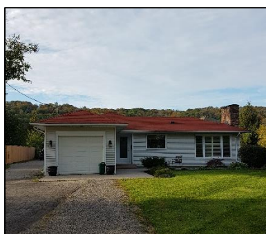
Figure 4: 226 Main Street East, looking south (ASI 2018)
