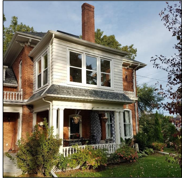
Figure 39: 224 Main Street East, east addition and east elevation
