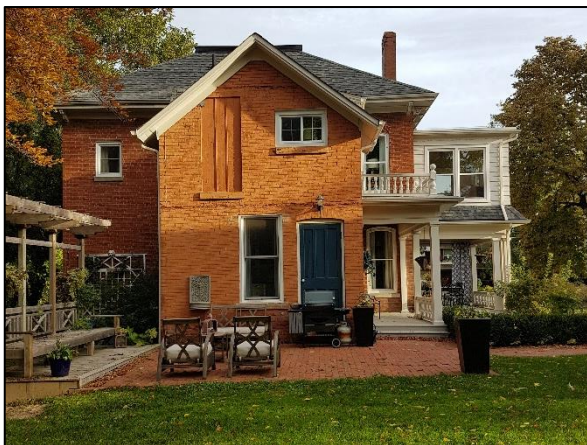
Figure 36: 224 Main Street East, showing rear (south) elevation
