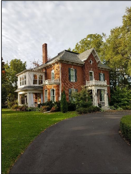
Figure 32: 224 Main Street East, showing the northeast corner and north elevation, looking southwest (ASI 2018)
