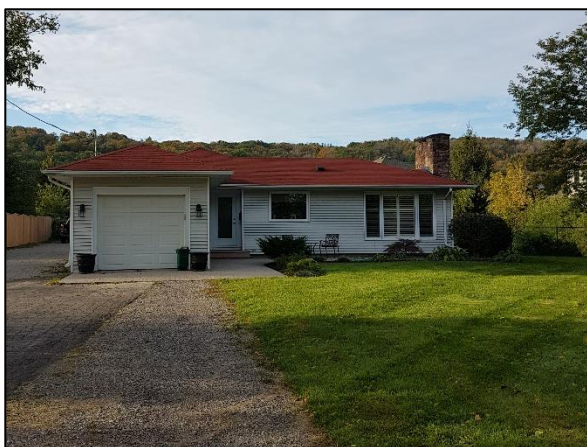
Figure 42: 226 Main Street East, showing front elevation of existing residence
