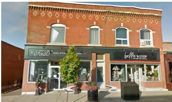
3 Main Street West, listed on the Town's Heritage Register (Google Earth).
