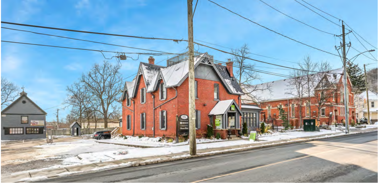
View of the Site looking southeast on Mountain Street. The Woolverton House at 13 Mountain Street is at the centre. A former Carriage House is located at the rear of the property (left). The Church (now in use as a community hall) at 19 Elm Street is at the right of the frame (photo courtesy of the property owner).
