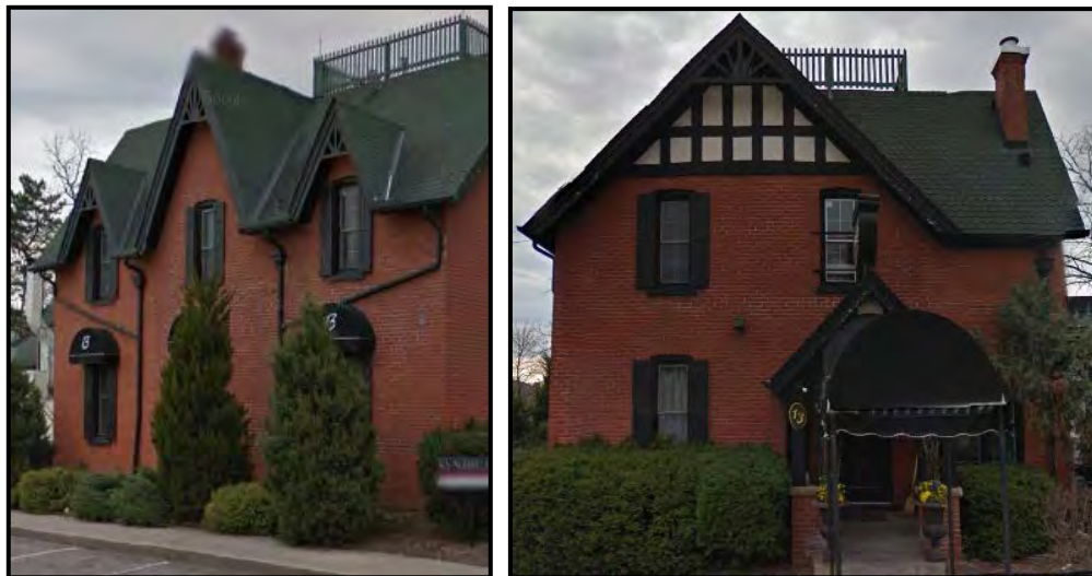
FIGURE 9: The three pitched gable roofline and narrow windows are signature features of Gothic Revival Architecture.
