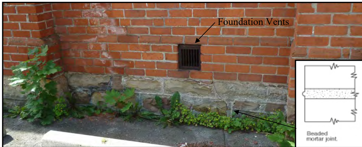
FIGURE 11: 19 Elm Street is a clay brick structure built on a stone foundation. The original foundation was arranged in a coursed layout with a cut stone and lime based mortar. The foundation mortar shown above has a beaded mortar joint. The face of the cut stone was left with a quarried finish. Pictured above you can also see the foundation vents which were used to keep the air circulating in the basement to prevent the spread mold and mildew in the summer months.
