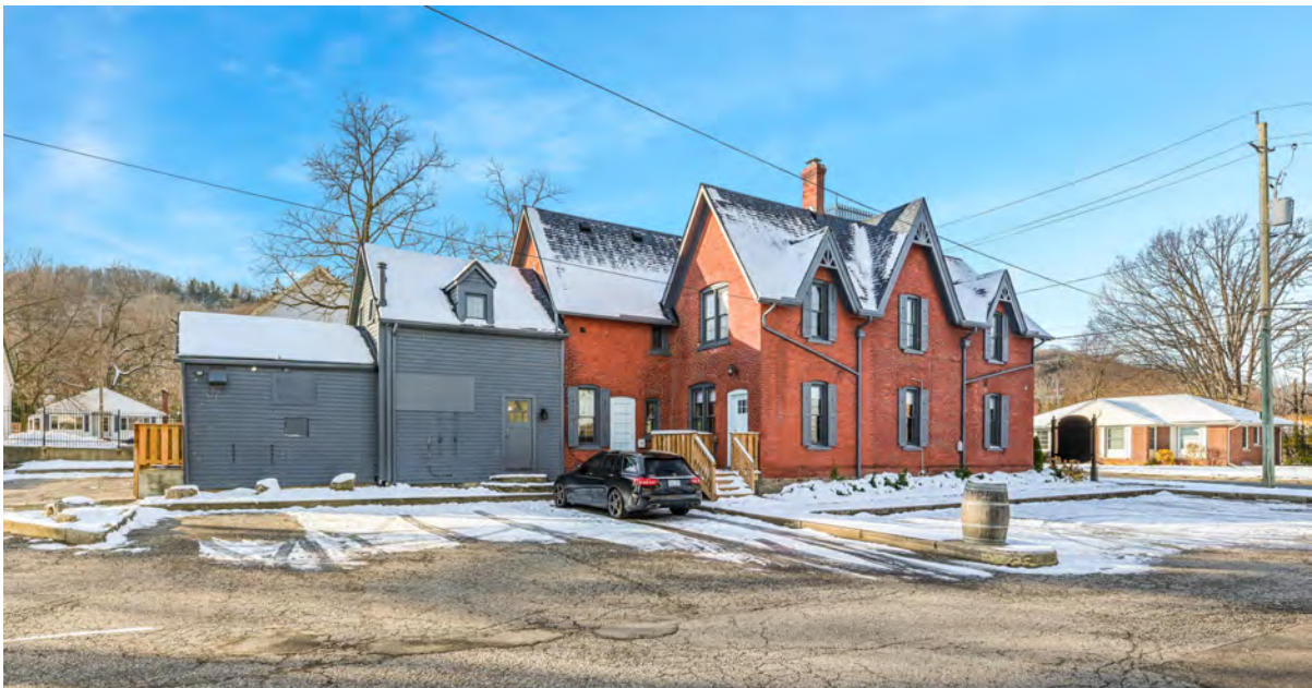
North elevation of 13 Mountain Street, showing part of the surface parking lot (photo courtesy of the property owner).
