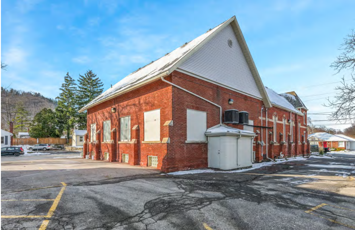
East and north elevations of 19 Elm Street, with view of the property's associated parking lot (photo courtesy of the property owner).
