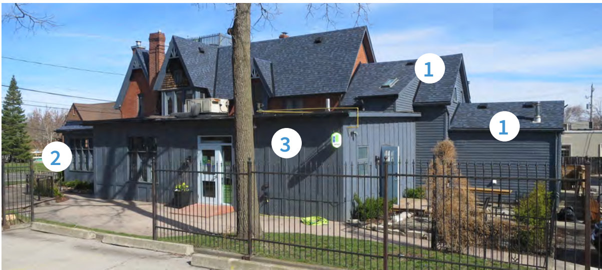
Views of the incremental additions on the house, including (1) the rough cast additions seen in the 1914 and 1928 fire insurance plans, (2) the enclosed sunroom from Lily Selby and Francis Woolverton's tenure beginning in 1933 and (3) a commercial addition from the late 20th century (ERA, 2021).
