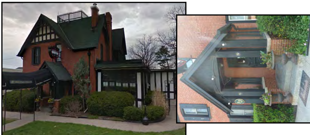
FIGURE 11: The portico seen on the front façade has a pitched roof structure that mimics the roof pitches above. The portico is supported by half columns resting on half walls made of brick that attach back to the front façade. The side porch was converted into a sunroom in the 1930s.
