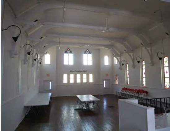
Present (2021) use of the church building as Woolverton Hall community space. View of the sanctuary space from the division between the 1880 building and the 1913 Sunday School addition. The far wall is the front (west) elevation of the church (ERA, 2021).
