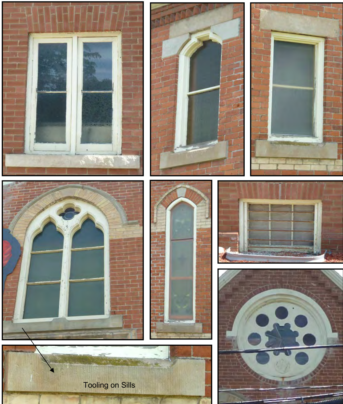
FIGURE 13: Pictured above are the original wood windows found throughout the exterior of 19 Elm Street. The sills and lintels on the above windows are cut stone with tooling details. On the new addition (after 1880) we can see the sills are cut stone without the tooling finish. The style of windows above include a rose window at center of front façade, above double lancet arch windows with a quatrefoil window in the center, lancet windows on nave of the church, and sash windows throughout.
