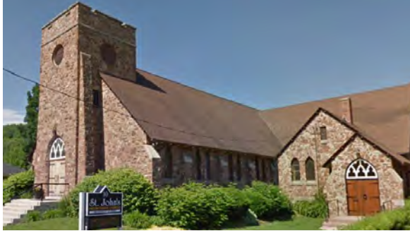
10 Mountain Street, listed on the Town's Heritage Register (Google Earth).
