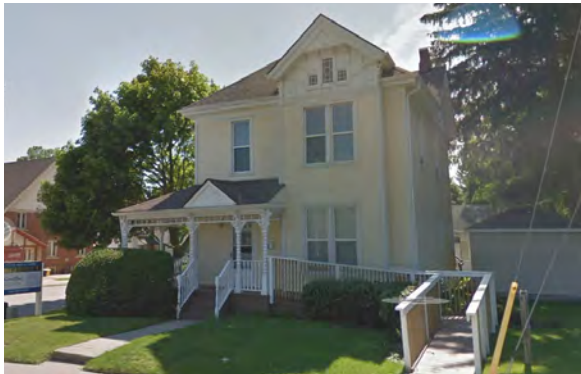
19 Mountain Street, listed on the Town's Heritage Register (Google Earth).
