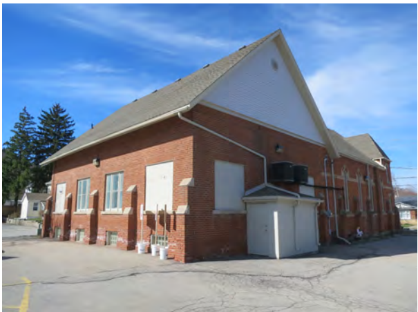
Current photo of the Church showing the east and north elevations of the 1913 Sunday School addition, which was designed with the same brick pier pattern as the original 1880 church. The north elevation of the addition was originally obscured by a drive shed, and is therefore unornamented (ERA, 2021).
