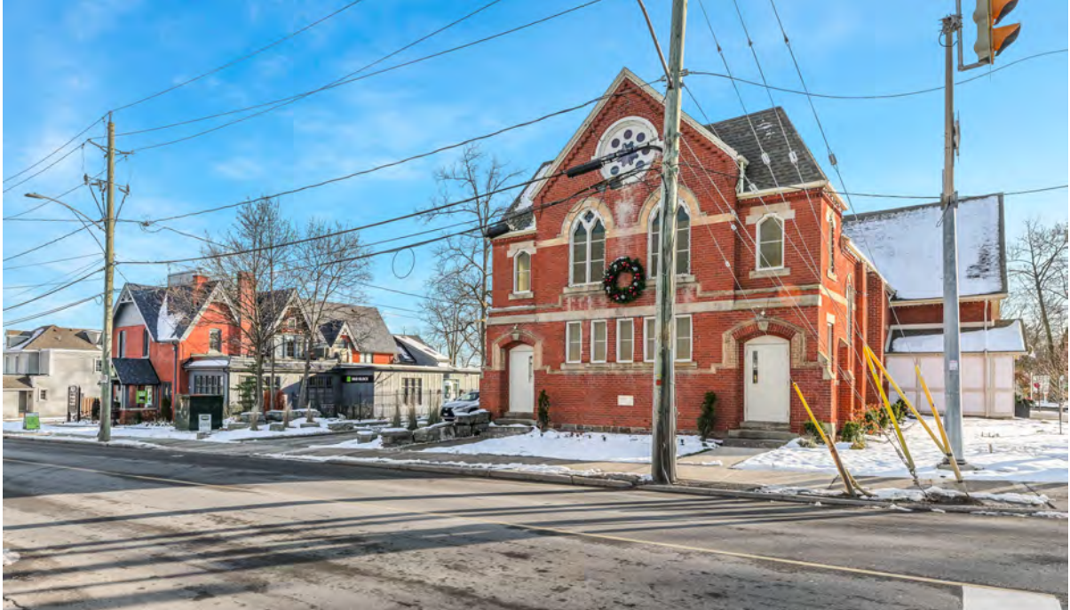
Mountain Street frontage of the Site, view east of the west elevation of 19 Elm Street (photo courtesy of the property owner).
