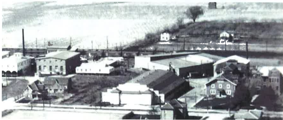
Dominion Cold Storage Facility and Grimsby Arena, Source Province of Ontario Archives
