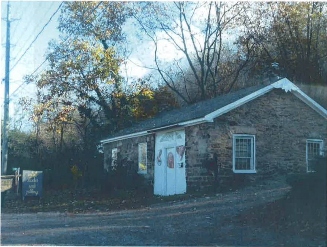
The Stone Shop (Alan Nixon Jr. UEL Blacksmith Shop), circa 1800
