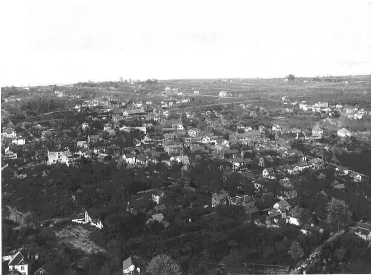
View towards Mountain Street Source Province of Ontario Archives
