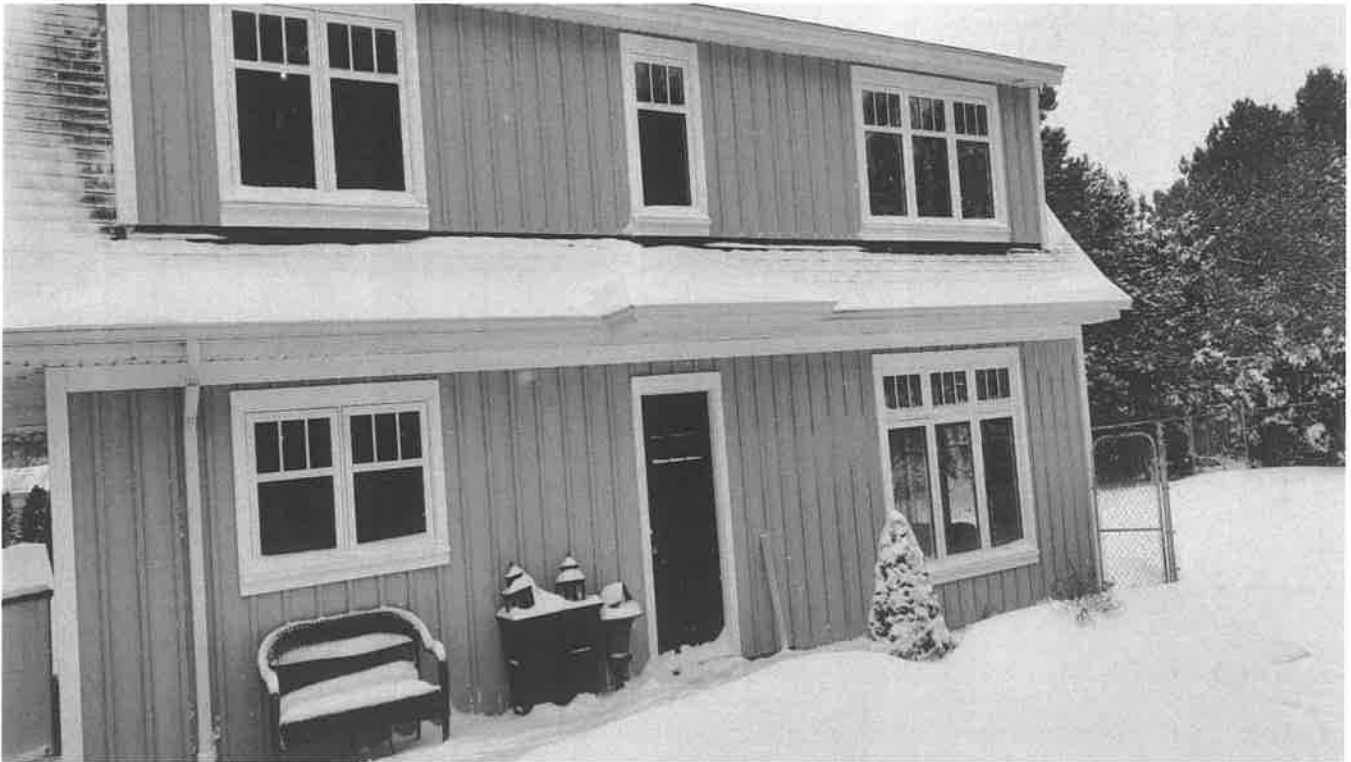
General view of the exterior of the residential structure at the subject site (looking East)
