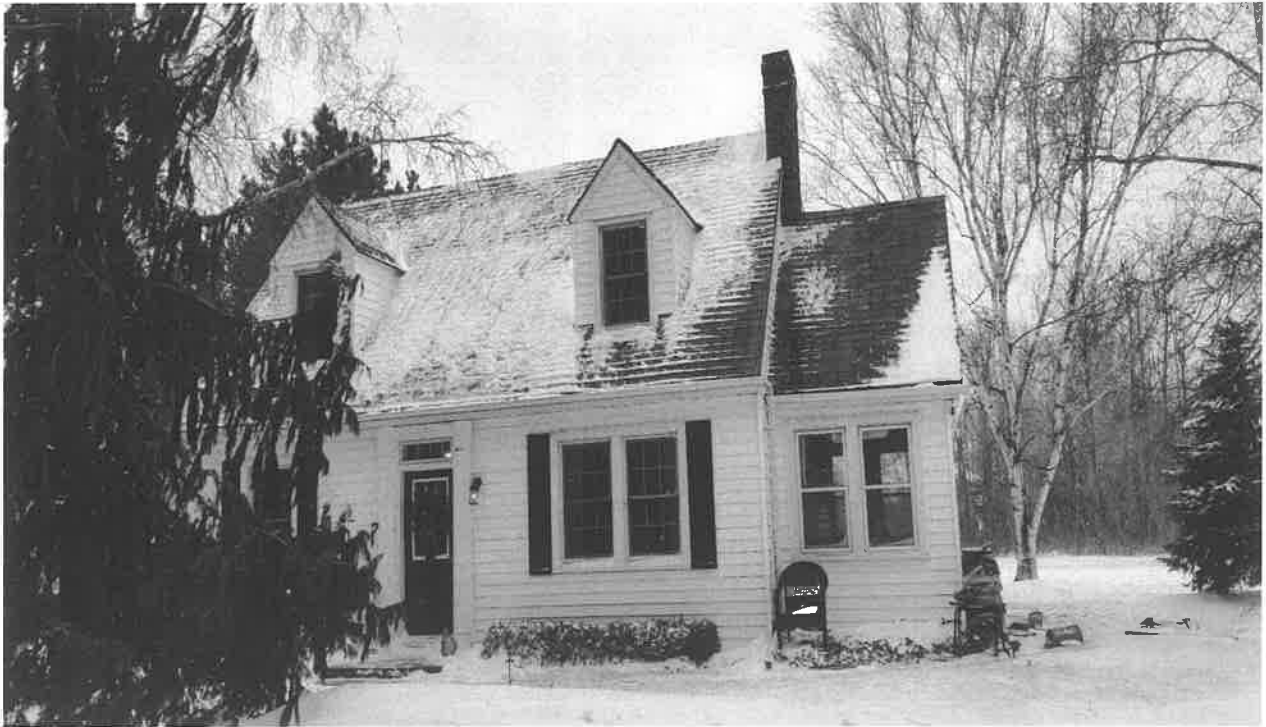
General view of the residential structure at the subject site (looking East)
