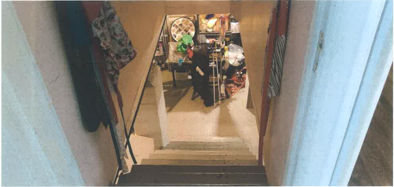
General view of the stairs to basement of the residential structure at the subject site
