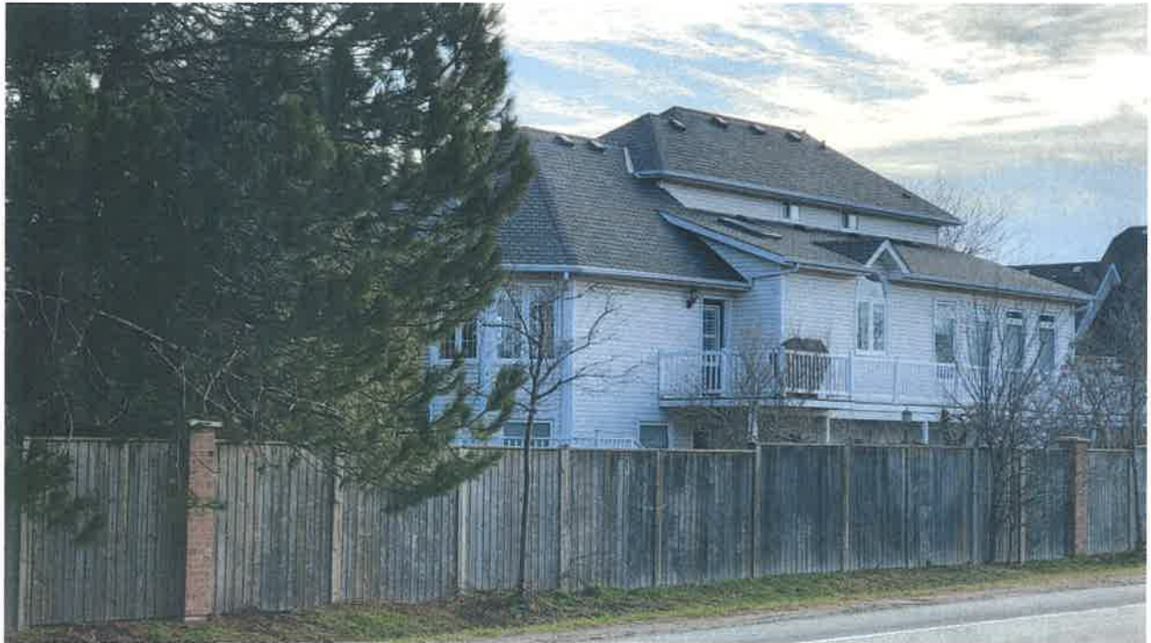
Neighboring properties to the east of the subject site (looking Northeast)
