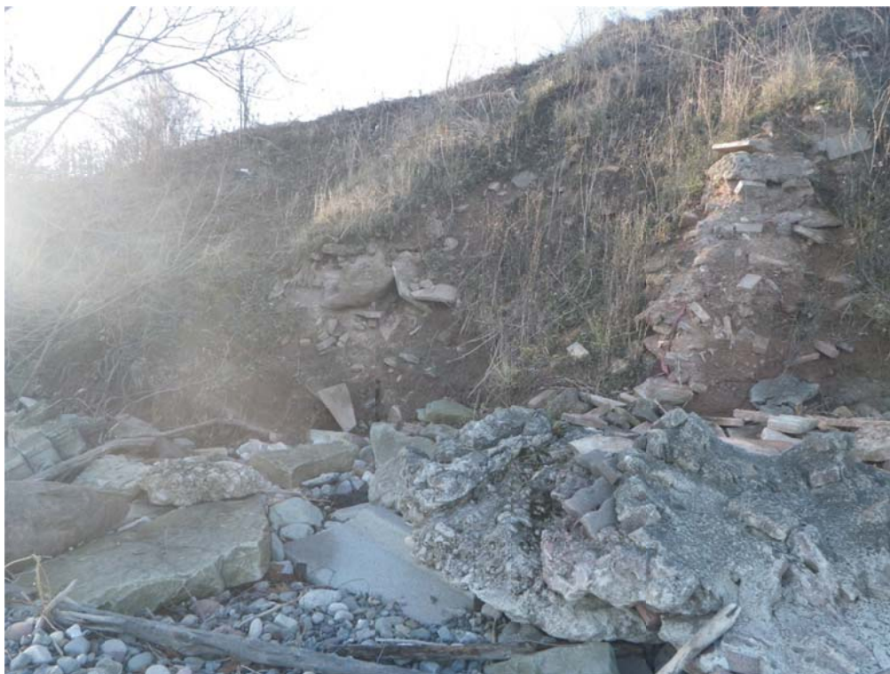
Photo 4 View of slope from shoreline
