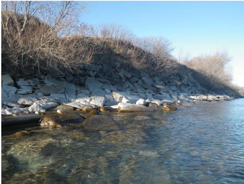
Photo 3 Shoreline at east end of subject site
