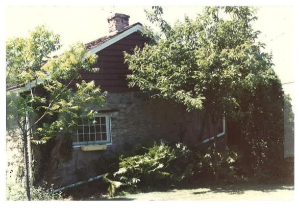
This facade is characterized by one fixed 18paned window with no trim. Unlike the other facades, this one has aluminum siding in the gable.
