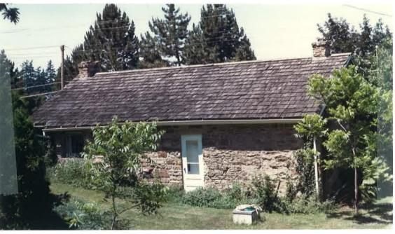
The South elevation is characterized by a center door with a fixed three upper section and a double paneled lower section. The window on this facade is a fixed twelvepane inset window. The roof line on this facade is extended an extra row of shingles above the window.
