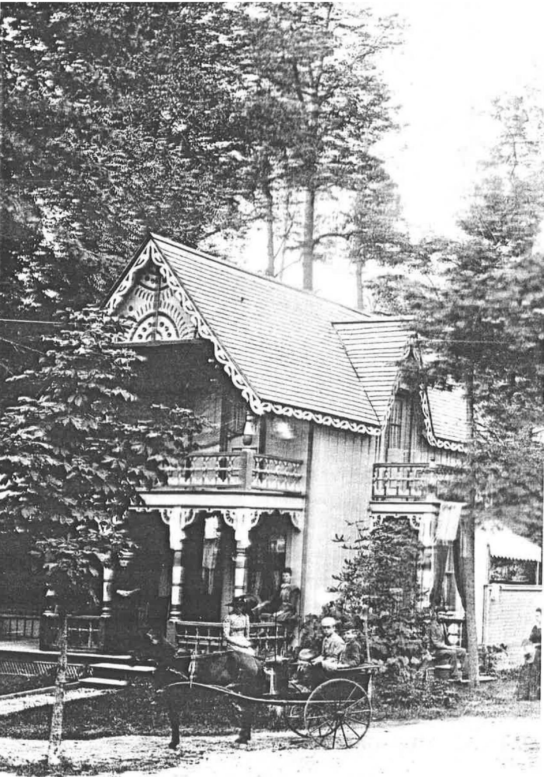
One of the "gingerbread" cottages that began to appear in 1875. Note the fretwork.
