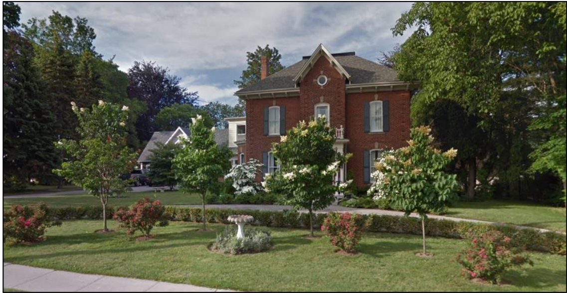
Figure 7 Front View of 224 Main Street East (“Udell House”), Grimsby, Retrieved from Google Street View 2017
