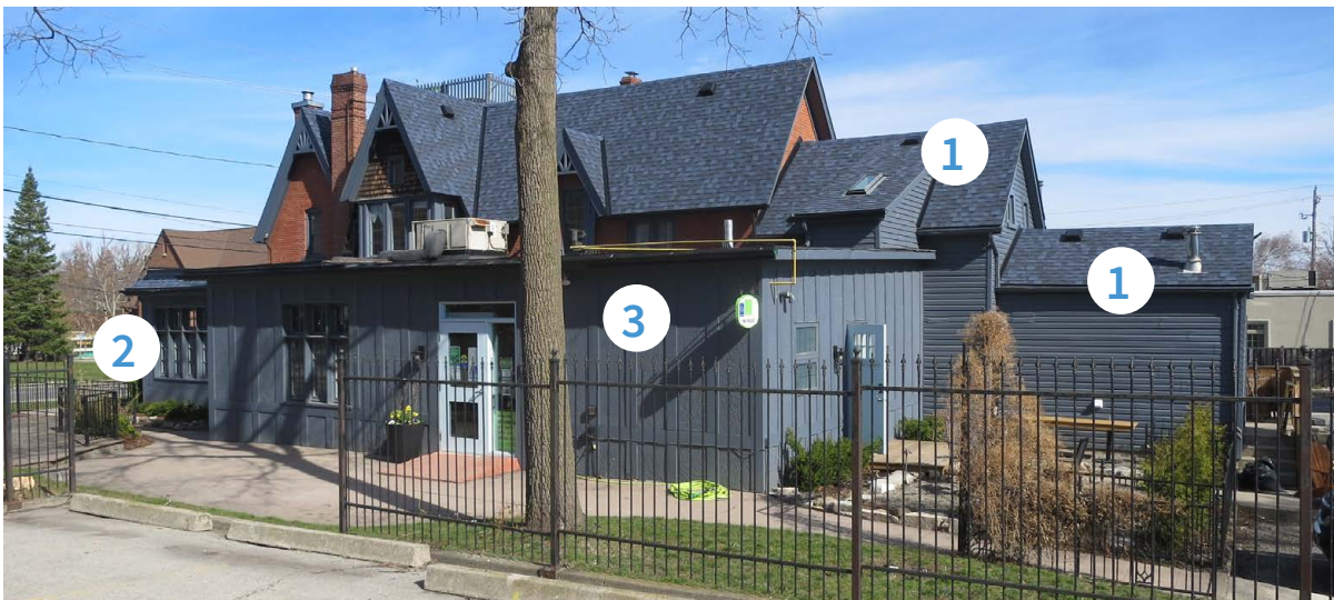
Views of the incremental additions on the house, including (1) the rough cast additions seen in the 1914 and 1928 fire insurance plans, (2) the enclosed sunroom from Lily Selby and Francis Woolverton’s tenure beginning in 1933 and (3) a commercial addition from the late 20th century (ERA, 2021).
