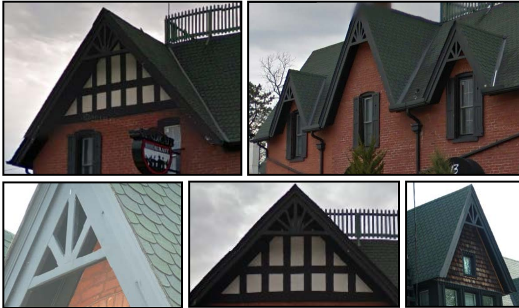
FIGURE 10: The high pitched gable roofs are decorated in gingerbread trim and accented with sections of half-timbering and cedar shakes. The pitched roofs and gingerbread trim are defining elements in gothic revival architecture.
