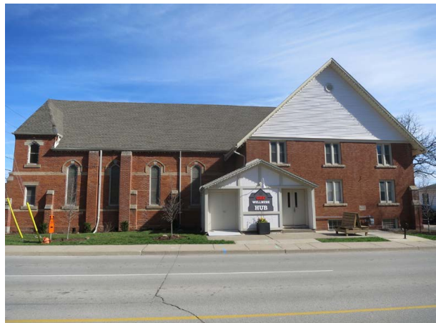
Current photo of the Church showing the south elevation of the 1880 Church (left), a later doorway addition (centre) and the 1913 Sunday School addition (right). The footprint and cross gable of the Sunday School addition somewhat obscures the original 1880 building footprint. The raised basement and first floor stand in contrast to the 1880 church building, whose first floor level sits much closer to grade (ERA, 2021).
