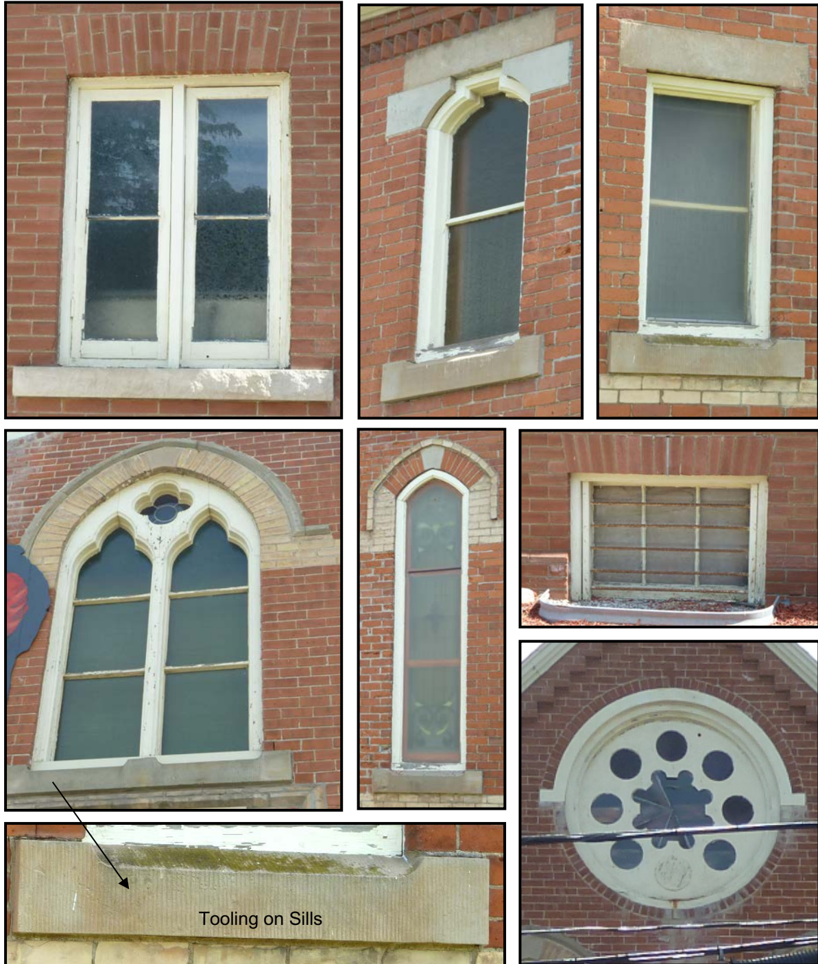
FIGURE 13: Pictured above are the original wood windows found throughout the exterior of 19 Elm Street. The sills and lintels on the above windows are cut stone with tooling details. On the new addition (after 1880) we can see the sills are cut stone without the tooling finish. The style of windows above include a rose window at center of front façade, above double lancet arch windows with a quatrefoil window in the center, lancet windows on nave of the church, and sash windows throughout.
