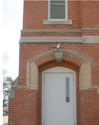
West elevation detail of northern doorway. Remove disused services (ERA, 2021).
