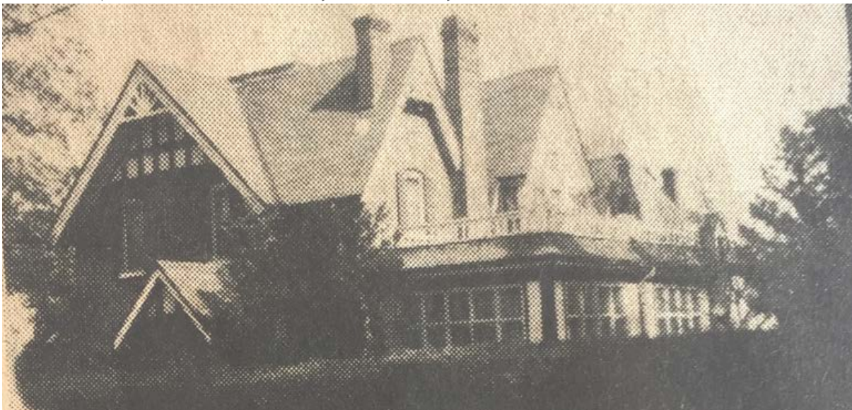
Undated archival photo of the Woolverton House after the south sun porch had been enclosed as a sunroom and the original front porch had been removed and replaced with a small gabled structure over the front door after the 1930s (Grimsby Archives).
