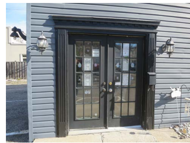
Modern window and door inserts and wood trim (ERA, 2021).
