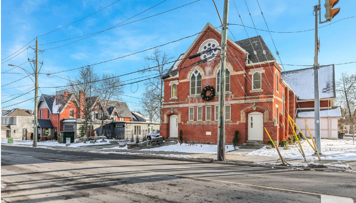
Mountain Street frontage of the Site, view east of the west elevation of 19 Elm Street (photo courtesy of the property owner).
