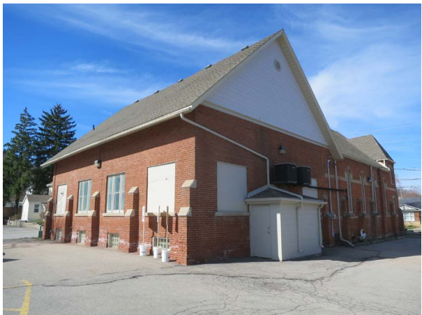
Current photo of the Church showing the east and north elevations of the 1913 Sunday School addition, which was designed with the same brick pier pattern as the original 1880 church. The north elevation of the addition was originally obscured by a drive shed, and is therefore unornamented (ERA, 2021).
