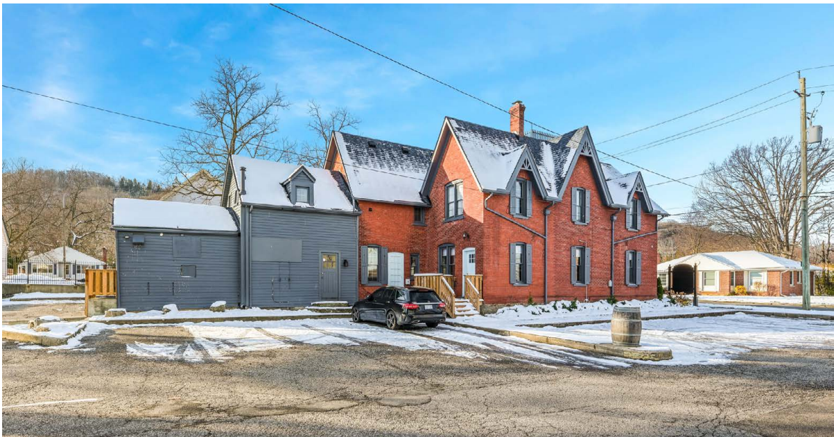
North elevation of 13 Mountain Street, showing part of the surface parking lot (photo courtesy of the property owner).
