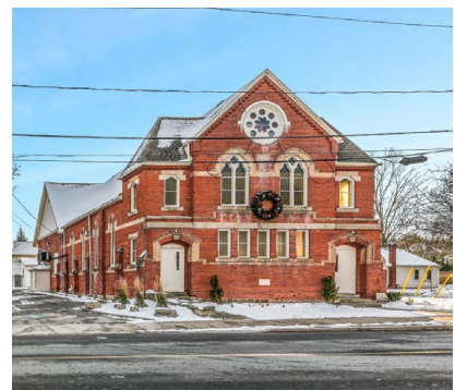
19 Elm Street, Mountain Street frontage (west elevation) (photo courtesy of property owner).
