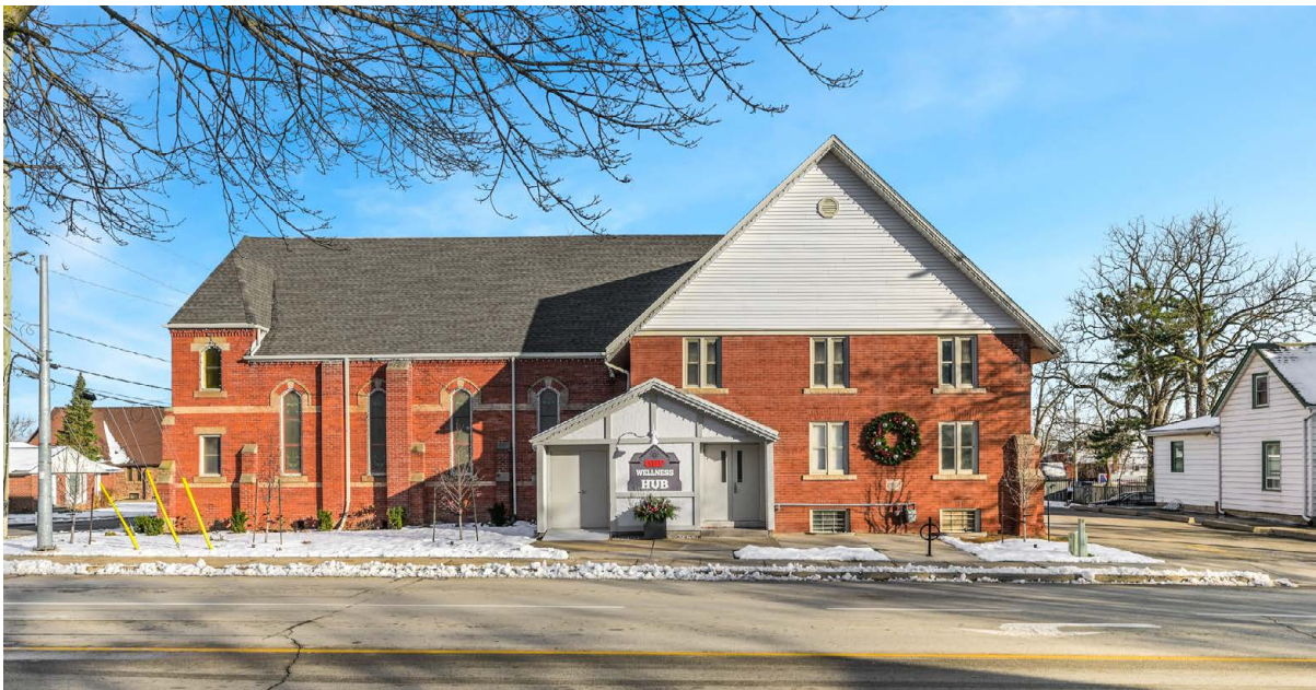
Elm Street frontage of the Site, view north of the south elevation of 19 Elm Street (photo courtesy of the property owner).
