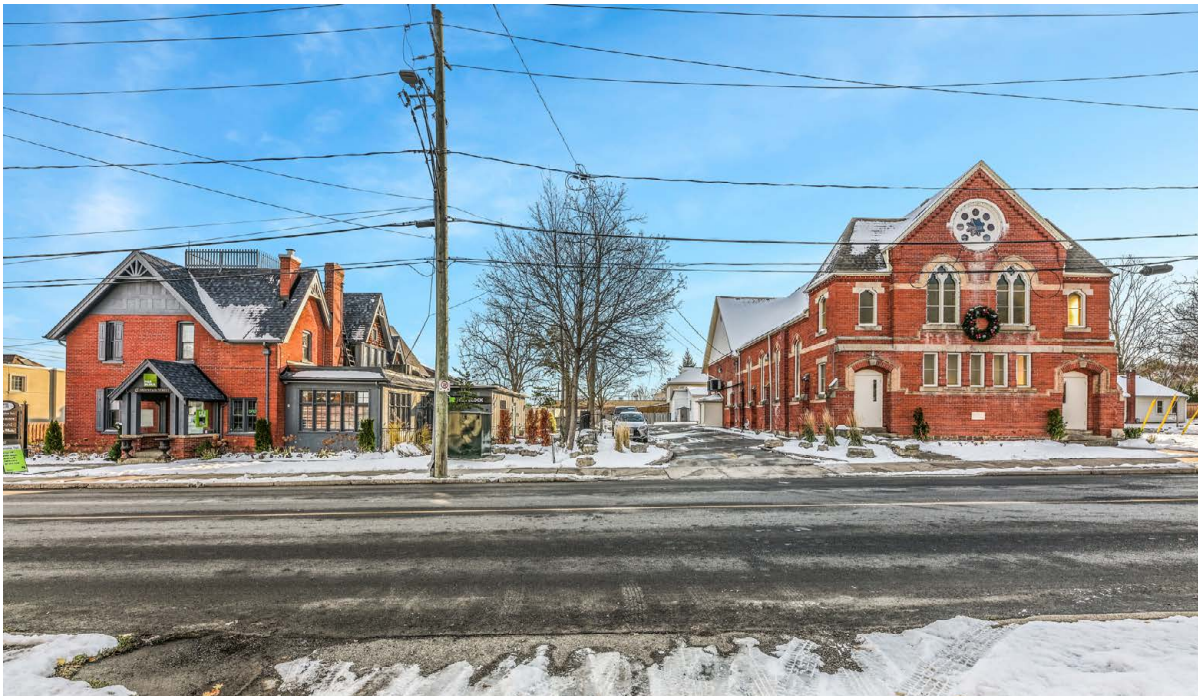
Photo of the Site from the west side of Mountain Street, view east. The west elevations of 13 Mountain Street (left) and 19 Elm Street (right) are pictured (photo courtesy of property owner).
