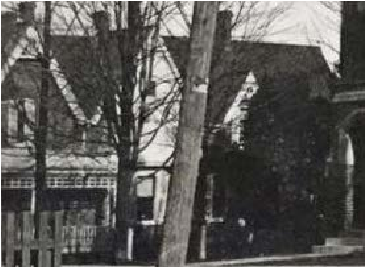
C. 1880 image showing the south elevation of the house at 13 Mountain Street. The original open sun porch with lattice structure can be seen, before it was later enclosed. This porch is shown to wrap around the front portion of the house in fire insurance plans from 1914 or 1928 (Grimsby Historical Society).
