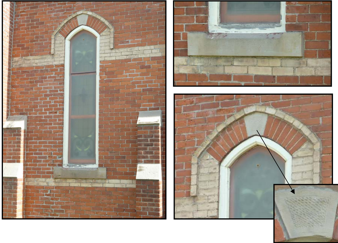
FIGURE 12: Pictured above are the original stain glass windows on 19 Elm Street. Donated by Linus Woolverton in memory of his father Charles Woolverton. The stained glass windows are designed in three panels that fit into wood frame surrounds, the original openings have had additional storm windows installed on the exterior side of the stained glass window with ventilation. The arch above the windows are constructed with; white clay bricks as the spring of the arch and red clay bricks as the voussoir's, the arch is then topped with a tooled key stone. The completed arch is then traced out with projecting headers in white brick. The sill under the stained glass windows are cut stone with tooling details. Throughout the structure white brick
