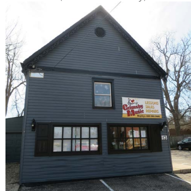
The former Carriage House has been altered, removing the original enlarged doors, recladding and the interior rehabilitation as a music school & store (ERA, 2021).
