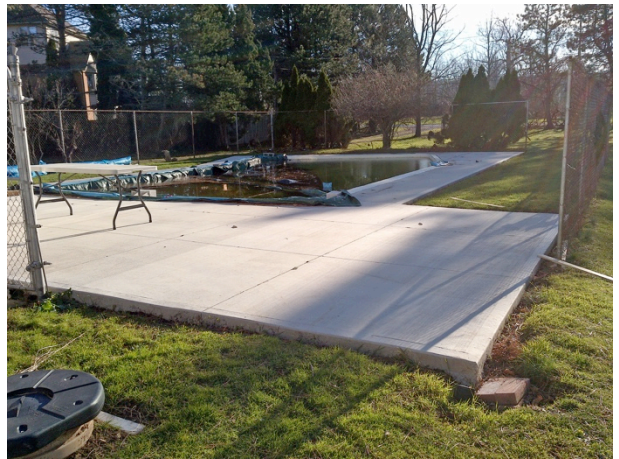
Plate 20: In-Ground Pool with Concrete Pool Deck
