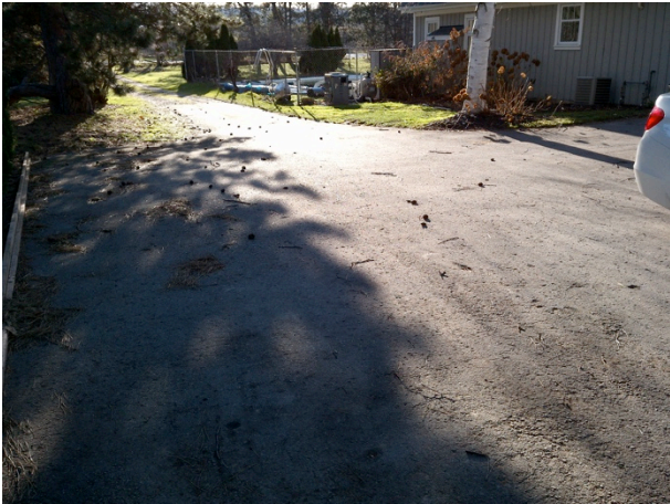
Plate 21: Asphalt Parking Area
