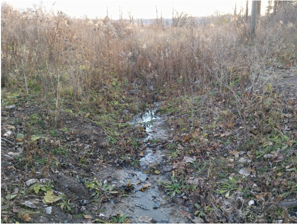
Plate 5: Landscaped Drainage Channel
