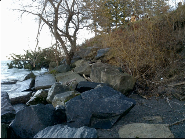
Plate 3: Rocks and Concrete Blocks for Shoreline Erosion Prevention
