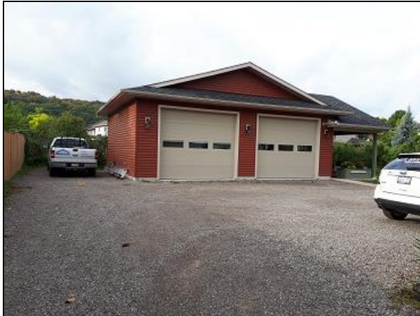
Plate 3: View of rear garage and gravel driveway in west half of property
