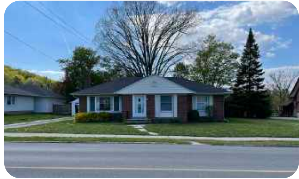
12 Elm Street, View looking west
