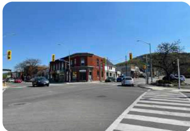
View looking southeast at the intersection of Mountain Street and Main Street West
