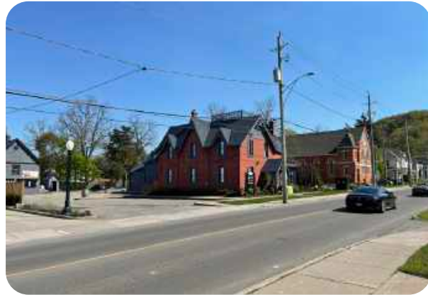
Subject Site, View looking southeast
