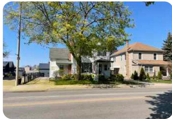
21 and 23 Elm Street, View looking north
