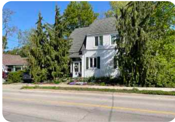
95 Main Street West, View looking east
