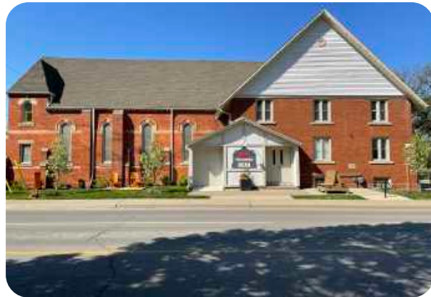
Subject Site - 19 Elm Street, View looking north
