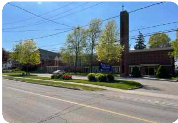
100 Main Street West (Trinity United Church), View looking west
