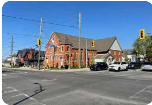
Subject Site, View looking northeast
