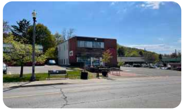
28 Main Street East, View looking southwest
