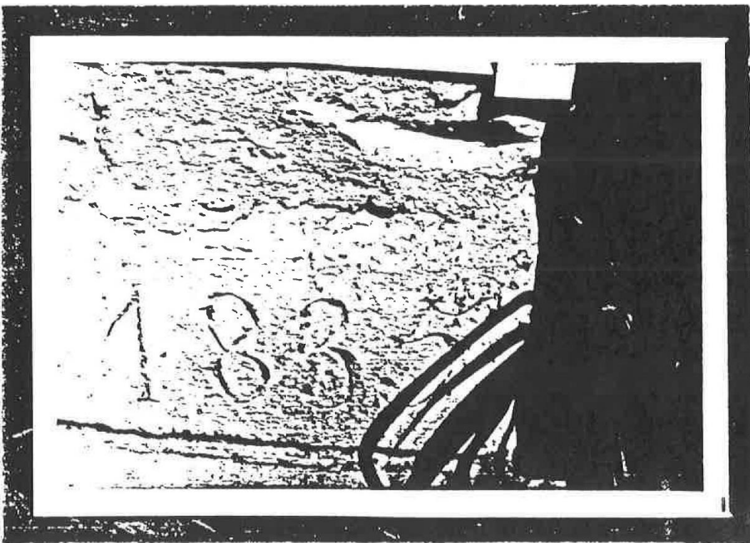
DATE FOUND ON SOUTH WEST CORNER OF EXTENSION WALL
