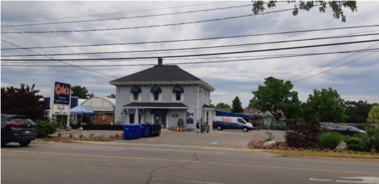
Figure 42 – View of front (south) elevation of 147 Main Street East, looking north (Source: Google Streetview, accessed 2020)
