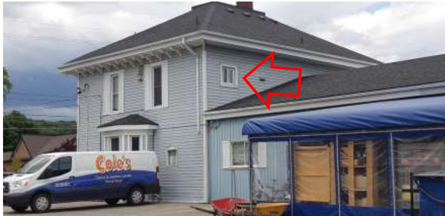
Figure 47 – View of rear (north) elevation of 147 Main Street East, looking west from Wentworth Drive. Location of square shaped window at north elevation noted with red arrow. (Source: MHBC, 2020)
