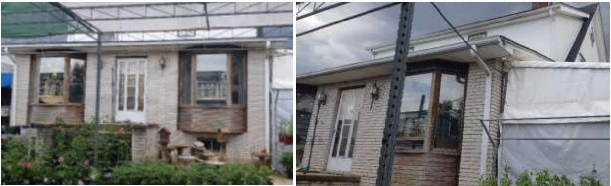
Figures 39 & 40 – View of north (rear) elevation addition, looking south, (right) View of rear elevation looking south-east from greenhouse/retail area (Source: MHBC, 2020)
