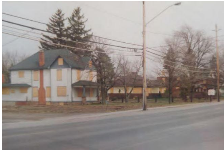
Pictured above are the demolished structures along Main Street East. Source: Grimsby Archives
