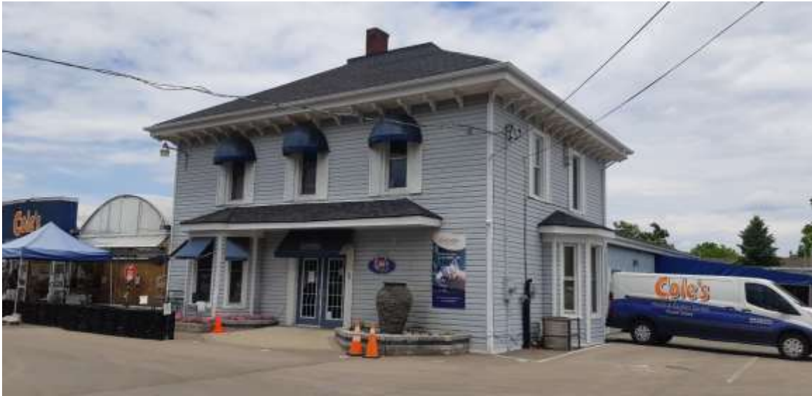
Figure 3: View of 147 Main Street, looking north-west. (Source: MHBC, 2020)
