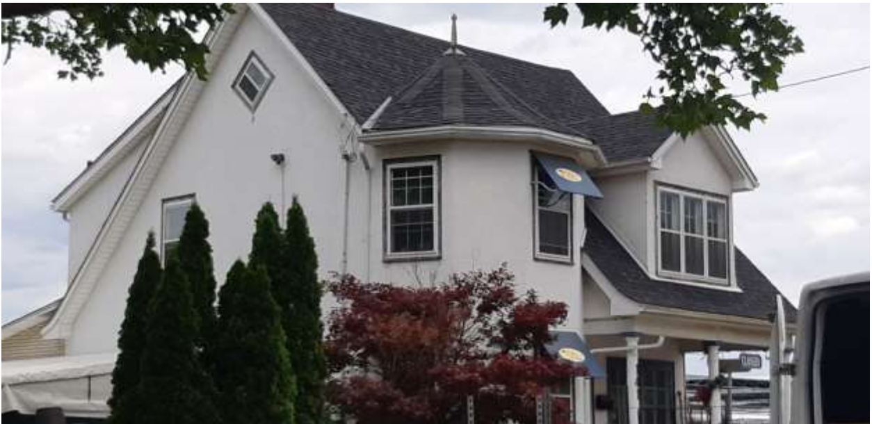
Figure 38 – View of front and east elevations looking north-west from parking lot (Source: MHBC, 2020)
