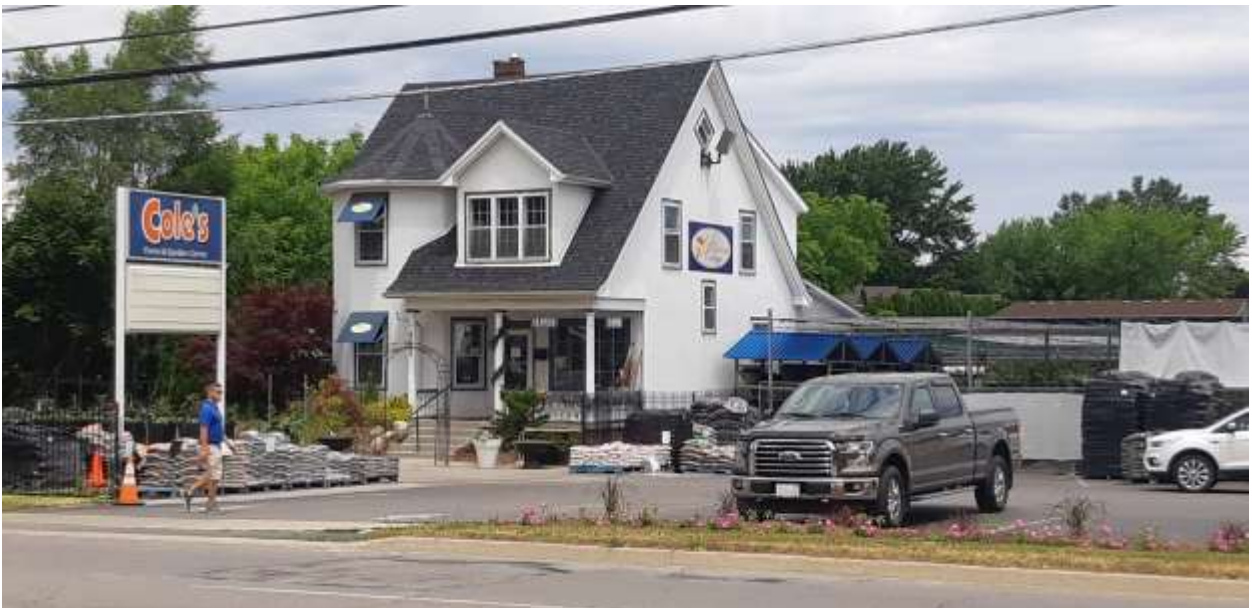
Figure 2: View of 141 Main Street, looking north-west. (Source: MHBC, 2020)
