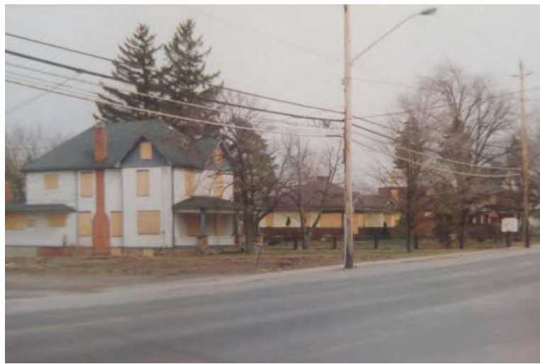
Pictured above are the demolished structures along Main Street East. Source: Grimsby Archives
