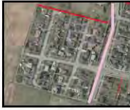
Residential Subdivision, Casablanca Boulevard and Livingston Avenue Built 1960s, fully serviced 36 Homes
