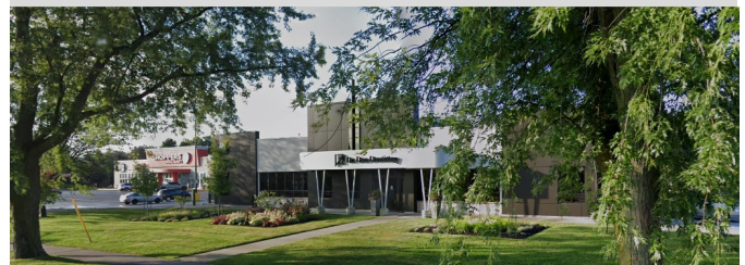
The south side of Main Street East is comprised primarily of commercial uses.
