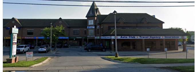
A two-storey commercial plaza (Orchardview Village Square) is located directly east of the subject lands.
