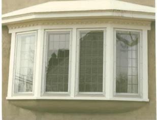
The North (side) facade features a four light bay light window with inset lower panels. A side entrance istopped by a neoclassical pediment supported by fluted pilasters. There are two single light over single light double hung windows equally distributed on the second floor. An architecture mold delineation the third floor which also exhibits a one over one double hung window. The neoclassical look of the north facade iscompleted with cornice returns.
