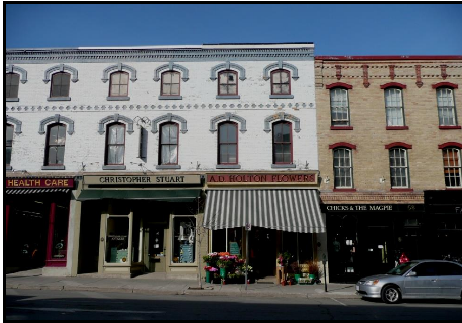
Figure 8: An image of restoration works in Port Hope, Ontario that represent good practice.
