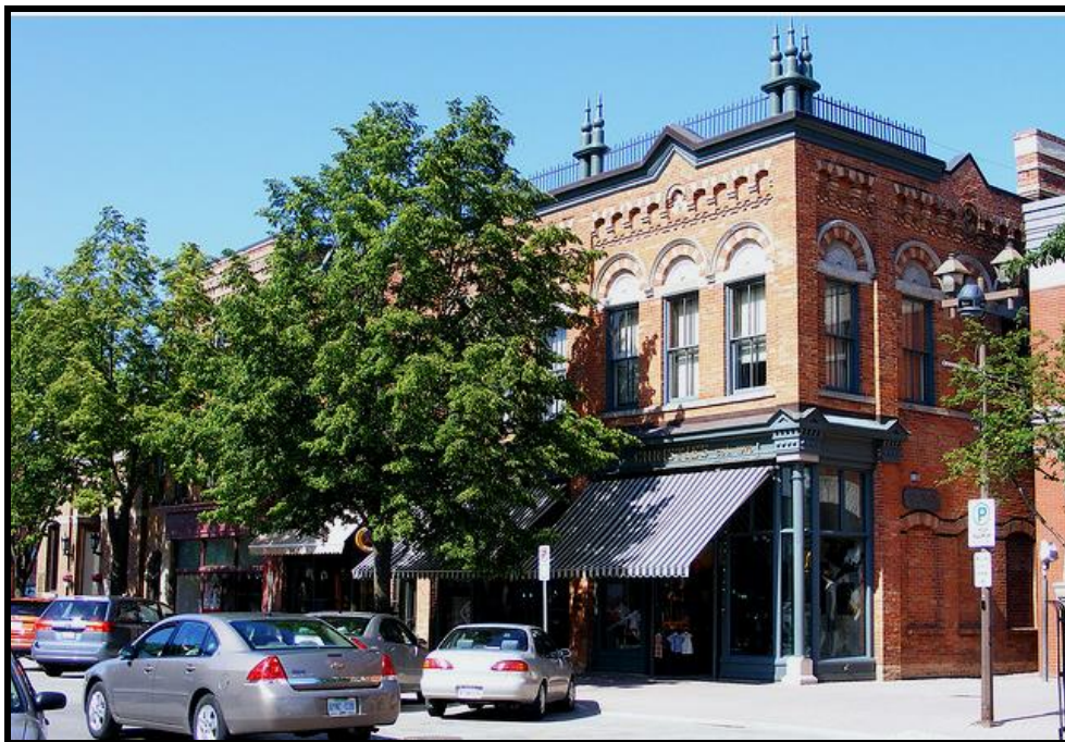
Figure 2: An image of a building in Collingwood, Ontario. The restoration works that this property underwent represent good practice.
