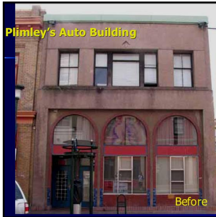
Figure 3: An image of a building in Victoria B.C before it underwent façade restoration works.
