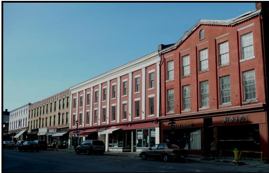
Figure 9: An image of restoration works in Port Hope, Ontario that represent good practice.
