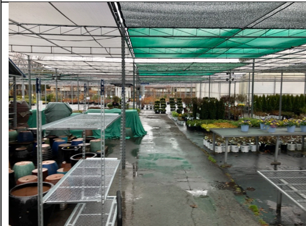
IMAGE 5 TEMPORARY STRUCTURES AND PAVED ASPHALT
