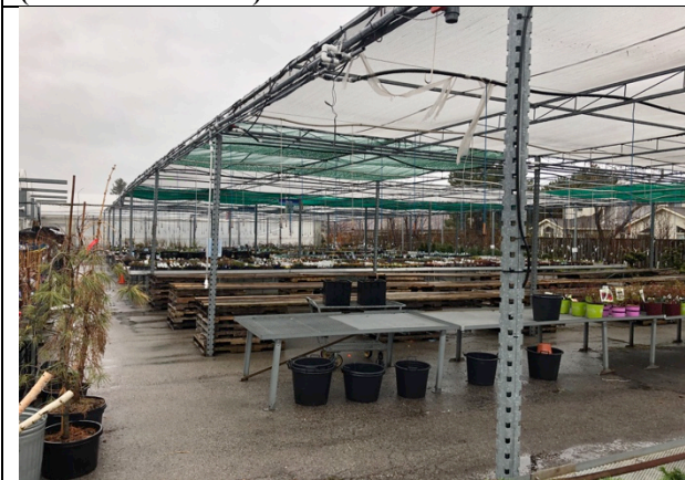
IMAGE 11 PAVED ASPHALT AND TEMPORARY STRUCTURES
