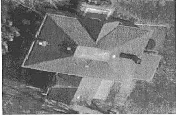
Figure 4 - Aerial Photo of Roof Structure
