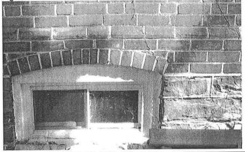
Figure 6 - Stone Foundation
