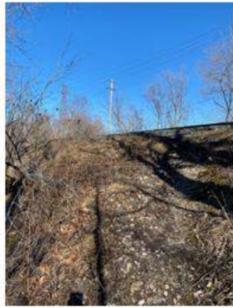
Unmitigated intersection of the trail and the rail line, evidence of desire line
