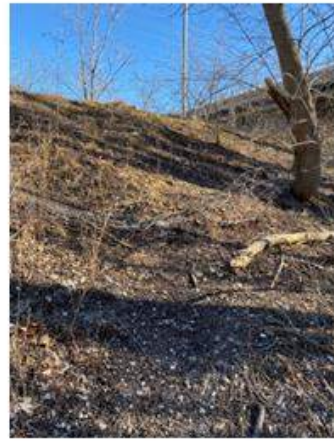
Trampled fencing at the intersection of the trail and rail line
