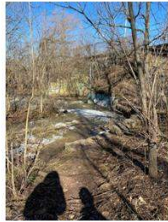
Forty Mile Creek tunnel beneath the rail line
