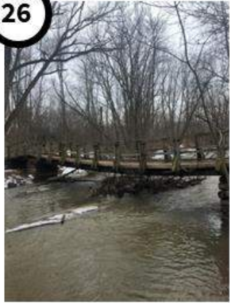
Existing Bridge crossing Forty Mile Creek south of Pumphouse
